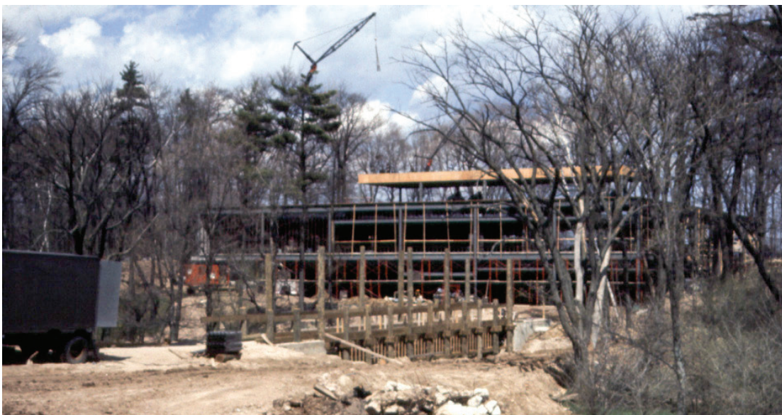
Left: The Bridge was constructed early to carry utilities from one side of the creek to the other.
